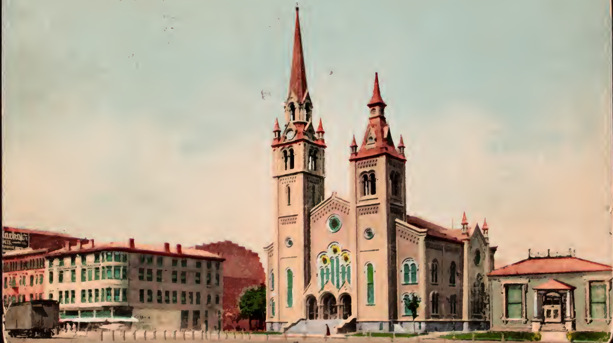
1627 - ELKS' BUILDING, ATHENIUM CLUB AND FIRST PRESBYTERIAN CHURCH. OAKLAND, CALIFORNIA.
